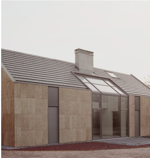
Sugar cane block construction
