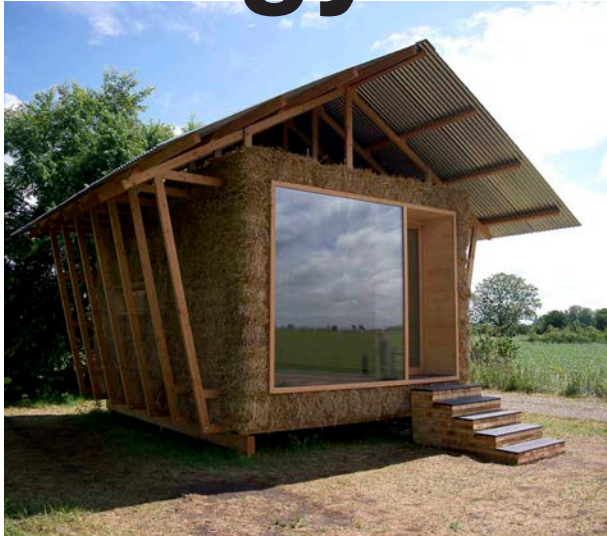
Sugar cane block construction
